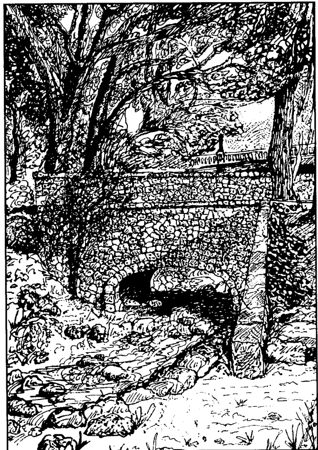
Stone Bridge at Live Oak Park
